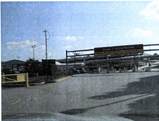
Entrance to Hourly Parking at BWI
