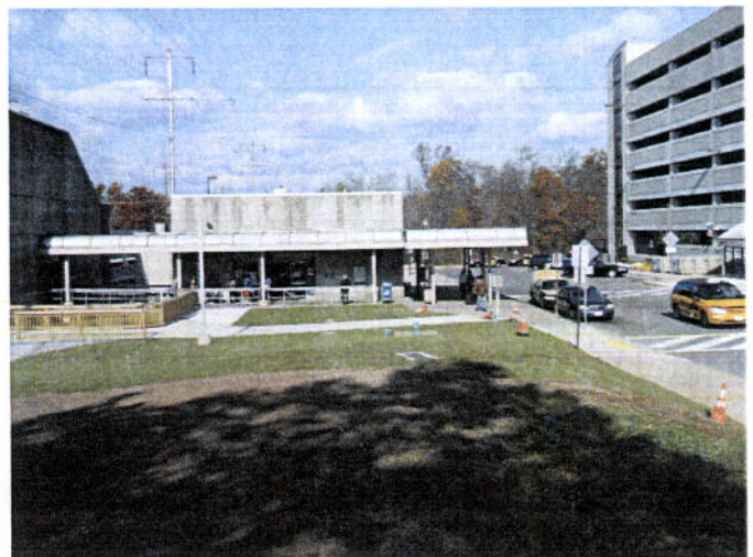
Amtrak Train Station with Parking to the Right
