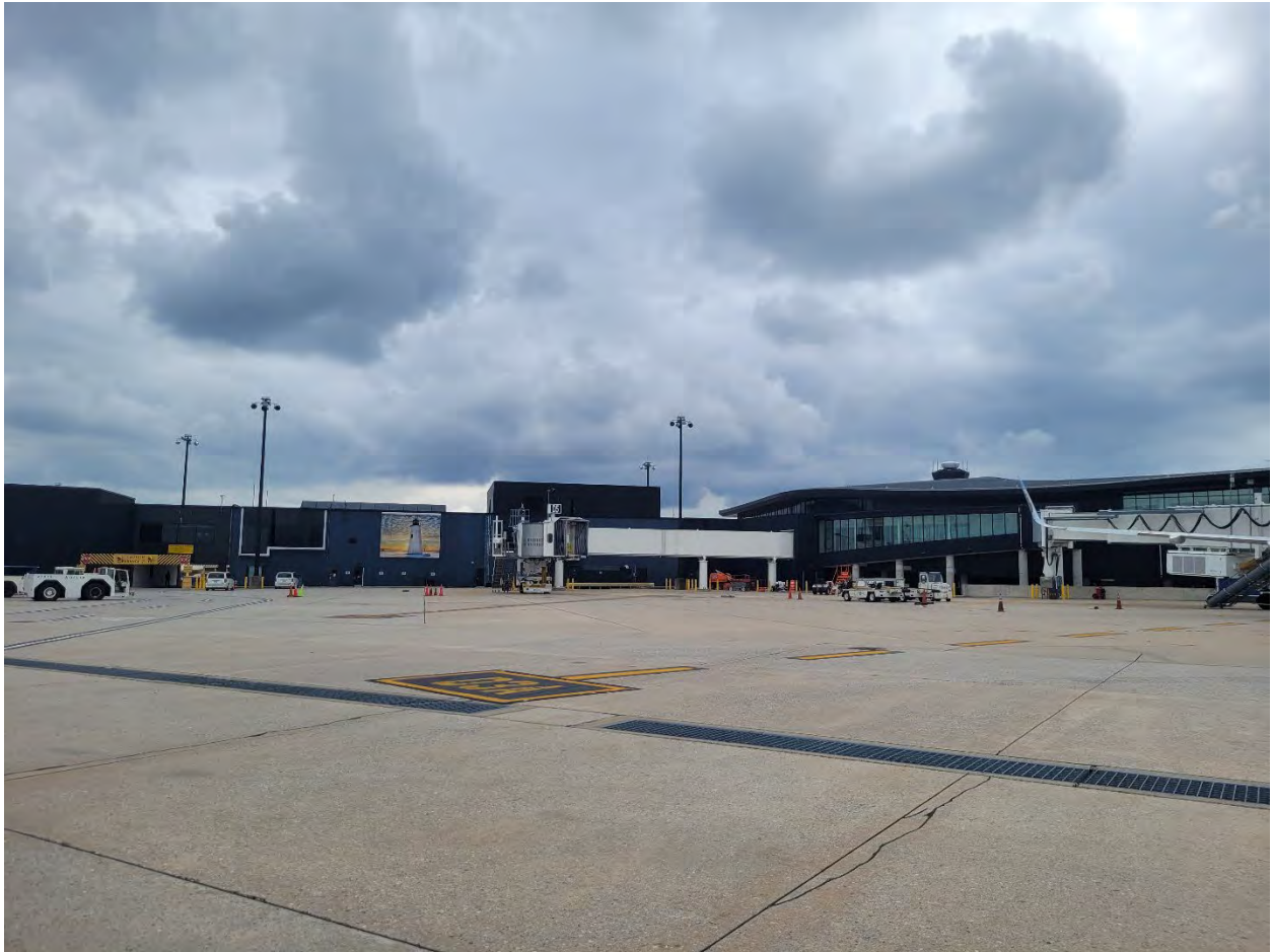
Photographic Plate 1: Proposed new ATCT location, facing southwest from between Concourses E and D
