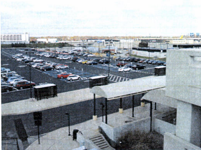
View from Hourly Parking Structure
