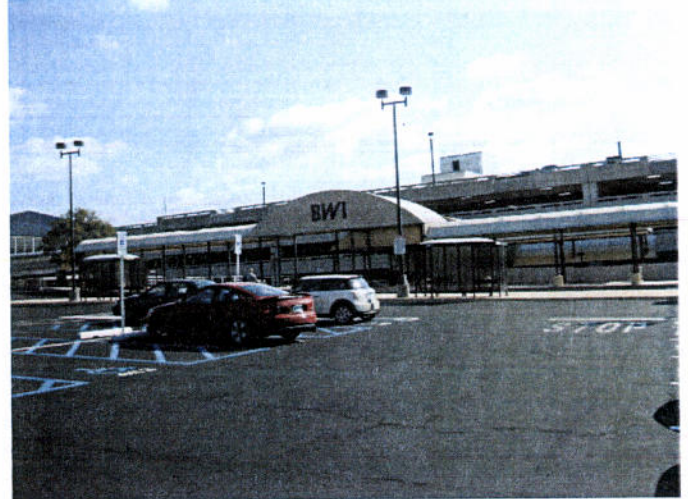
View of Hourly Parking Garage from Lot
