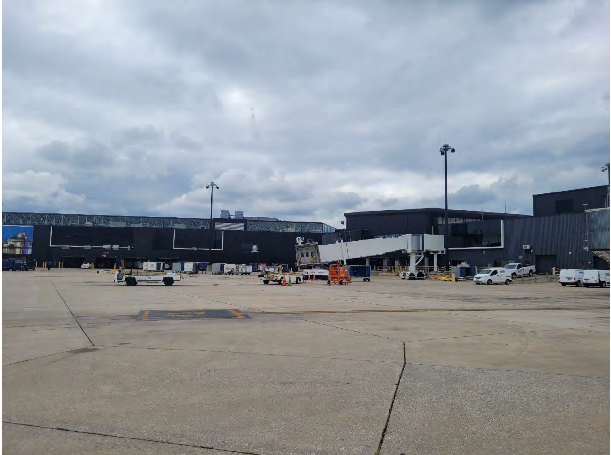
Photographic Plate 3: Proposed new ATCT location, facing northeast from between Concourses C and D
